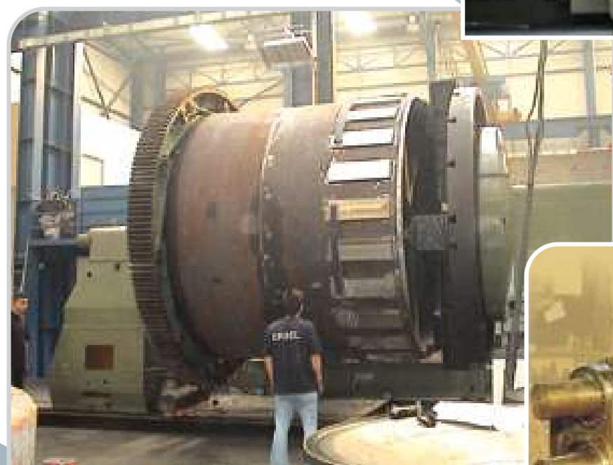
KILN SHELL UNDER TIRE
